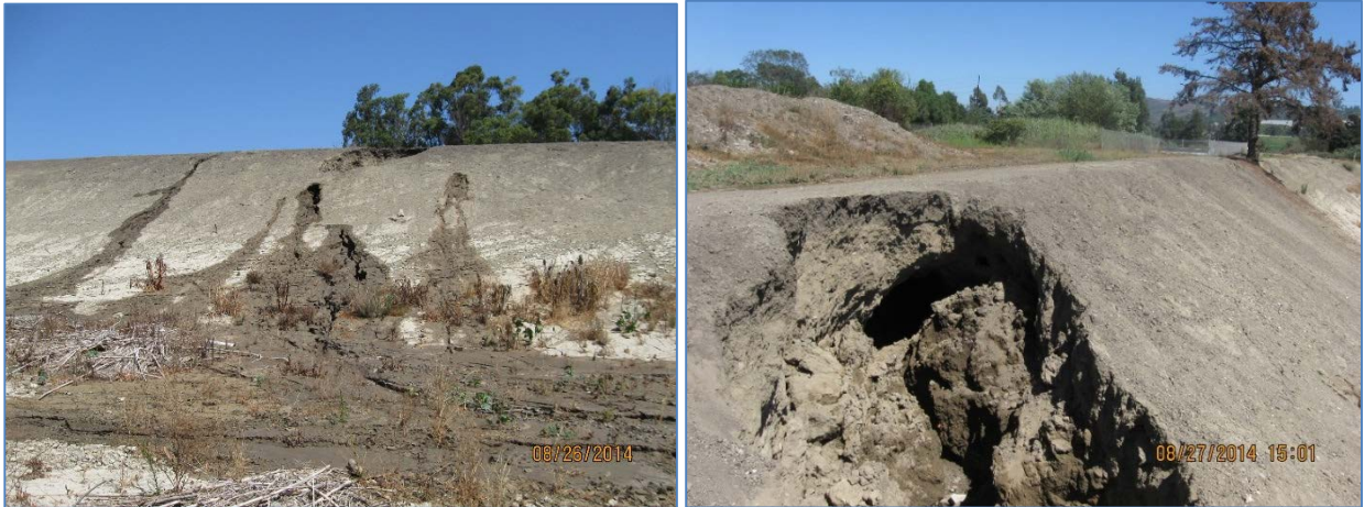
Figure 2. Fox Debris Basin “Piping” Damage as a Result of Seepage through Rodent Burrows
