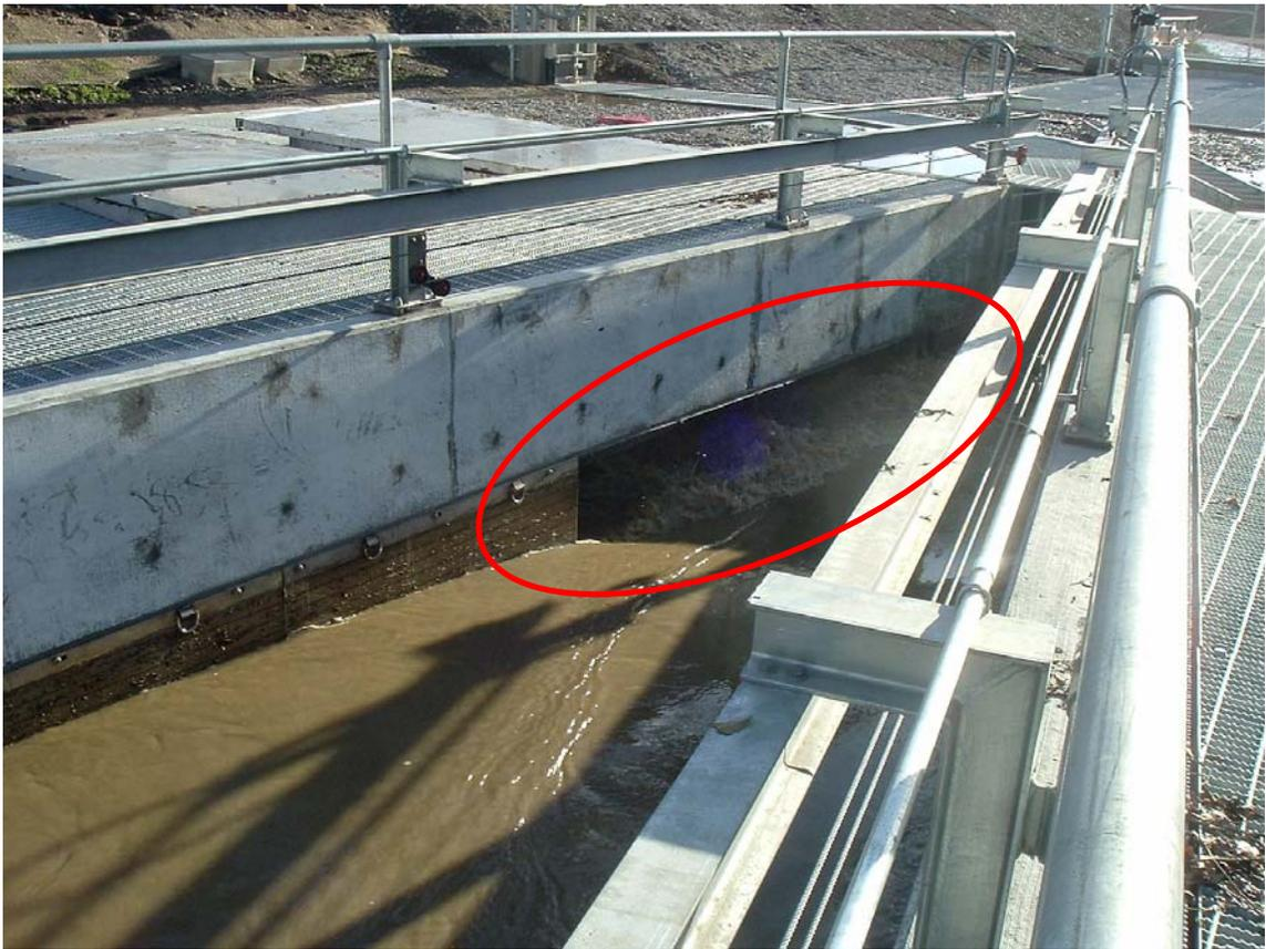
Figure 4.7. Picture Taken During January 2005 Flood Showing Fish Screens Removed in Robles Canal.
