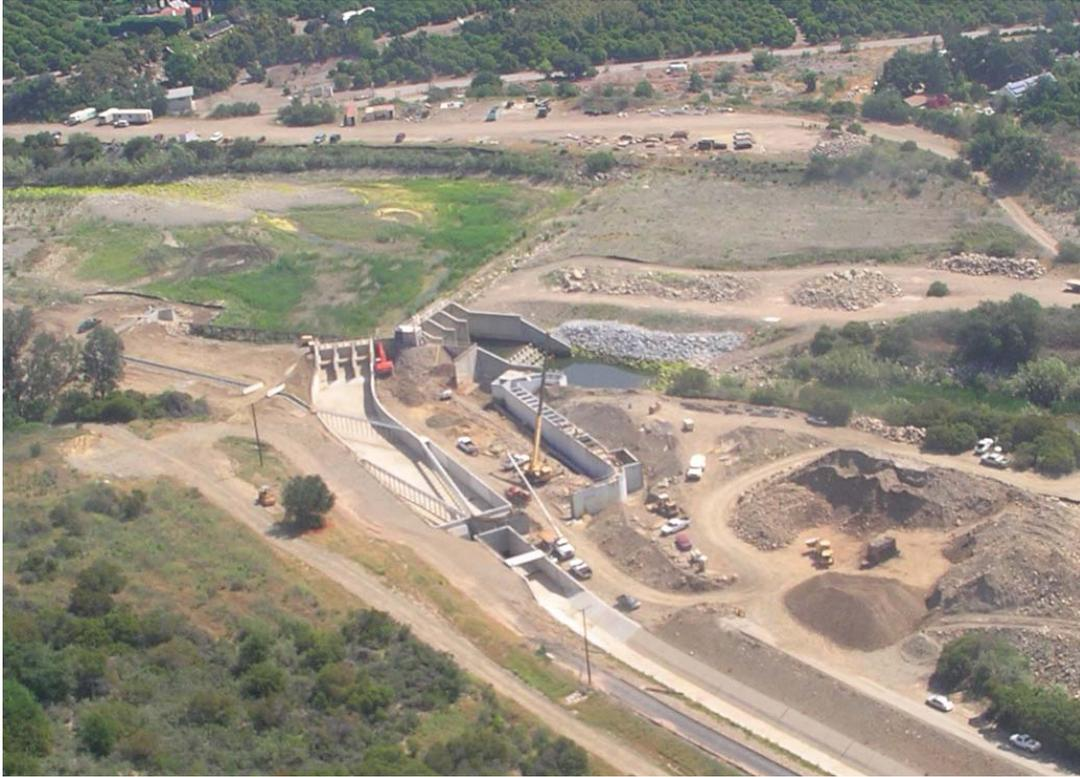
Figure 1.11. Aerial View of Robles Diversion Fish Passage Facility under Construction in April 2004.
