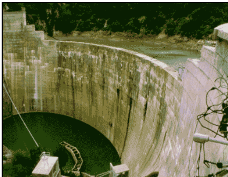
Figure 2. Matilija Dam After Notching
