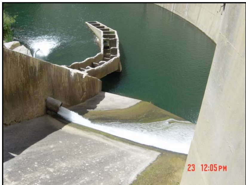
Figure 3. Fish Ladder Below Matilija Dam
