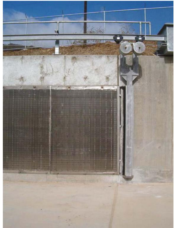
10/1/04 – Project construction continuing with the installation of fish screens and brush system. Note that the electrical and programming systems for the brush system were not installed until the last week of December 2004.
