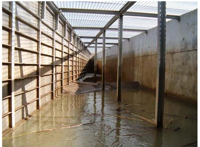
3/03/03 – District performed maintenance on the fish passage facility. Sediment deposition in the forebay.
