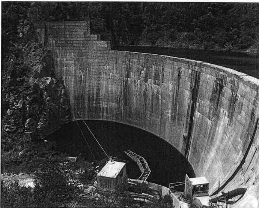
THE MATILAJA Dam, near Ventura, California, has already been notched to increase the stability of the structure, but sediment has nearly filled the reservoir and eliminated any flood protection potential.
