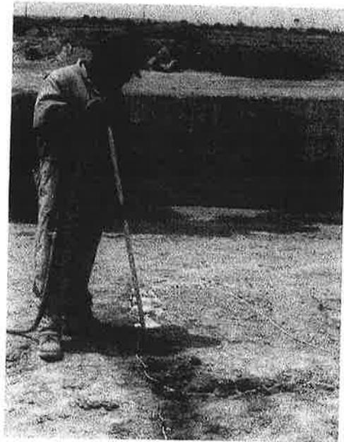
*Loading B-Gel into the holes after the detonating cord is simple and easy*
