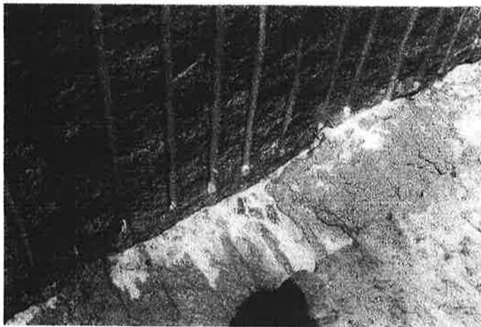
*Using B-Gel and detonating cord, much thinner slabs can be trimmed from a block than is possible by wedging. The natural shock absorbing properties of the gel leave corners square and undamaged.*
