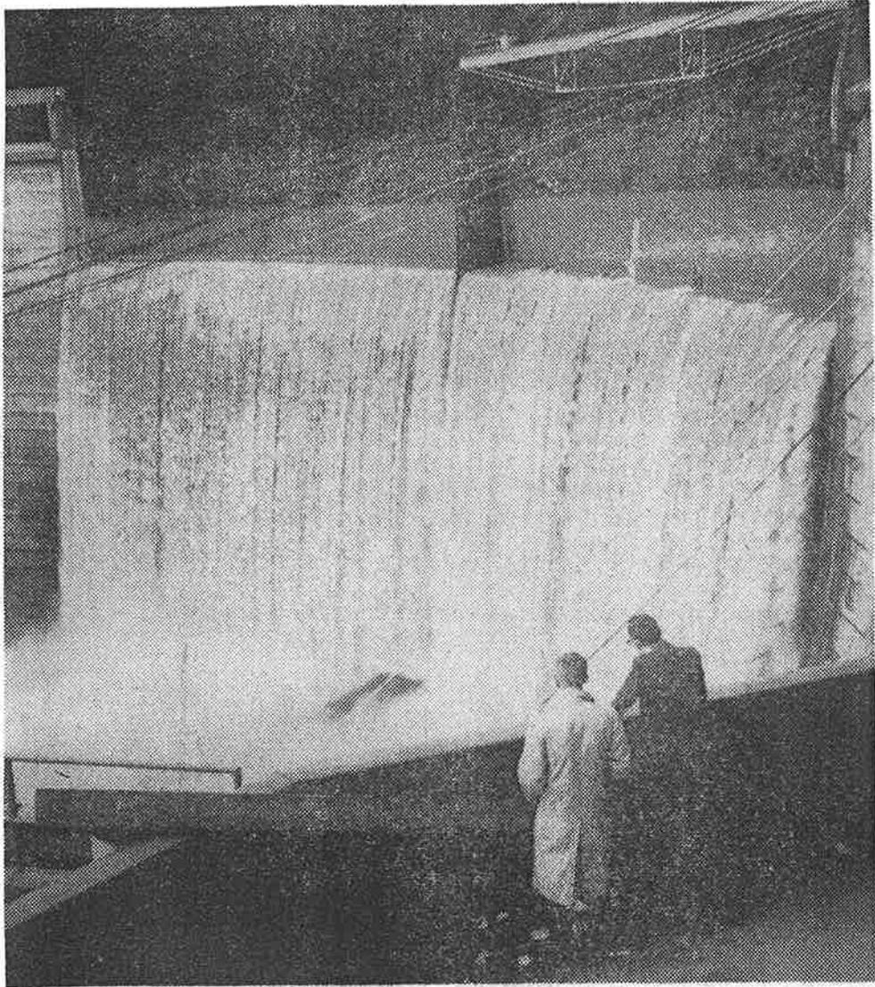
**OVER THE TOP** — The Matilija Dam northwest of Ojai, nearly empty last night, began spilling water this morning at 3 a.m. when a cloudburst hit the area. The water spilled over the notches cut in the dam late last summer to insure that the dam would be safe.
