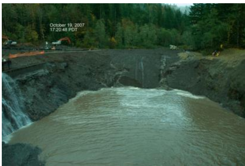
Figure 4.3-4. Photographs of the Sandy River Marmot Dam site (courtesy of Bruce McCammon) showing flow beginning to erode the cofferdam and the reservoir deposit.
