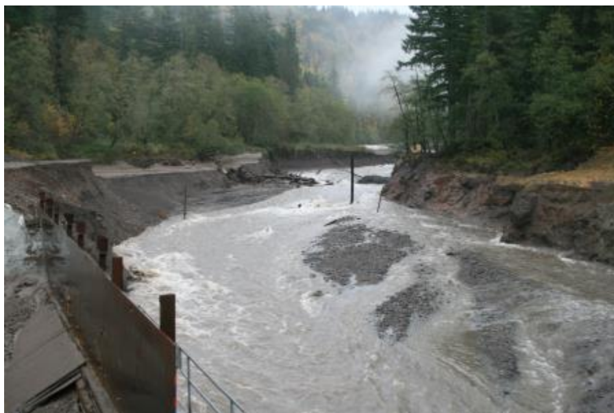
Figure 4.3-5. Photographs of the Sandy River Marmot Dam site (courtesy of Jon Major) approximately 13 hours after breaching, at which time the river appeared to be close to its natural conditions (ignoring the concrete and steel bars and plates on-site)
