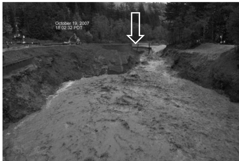
Figure A-4. Photograph of Marmot sediment deposit erosion approximately 20 min after the cofferdam was breached at a discharge of approximately 50 m 3 /s (1,750 cfs), showing the quick erosion of the cofferdam and the sediment deposit. The arrow points to the remaining portions of the cofferdam; flow direction is towards the camera (image courtesy of Bruce McCammon and US Forest Service).
