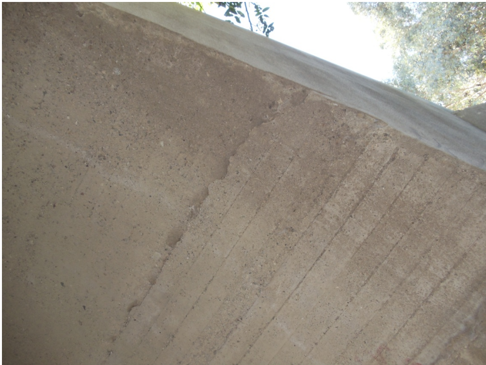
4 Longitudinal Construction Joint at Upstream Headwall
