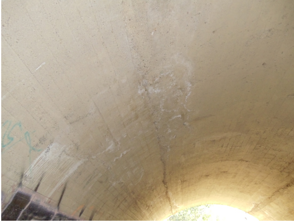
3 Longitudinal Construction Joint in Arch
