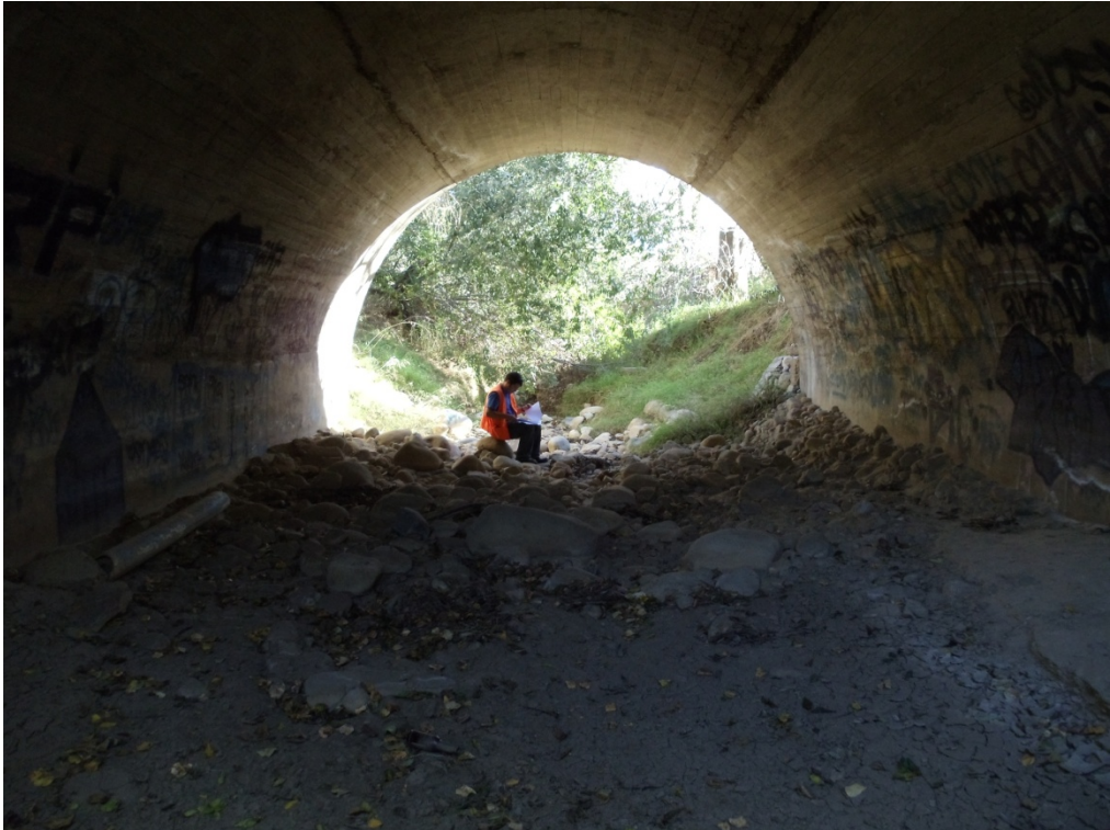
2 Unreinforced Concrete Arch Culvert (Looking Downstream)
