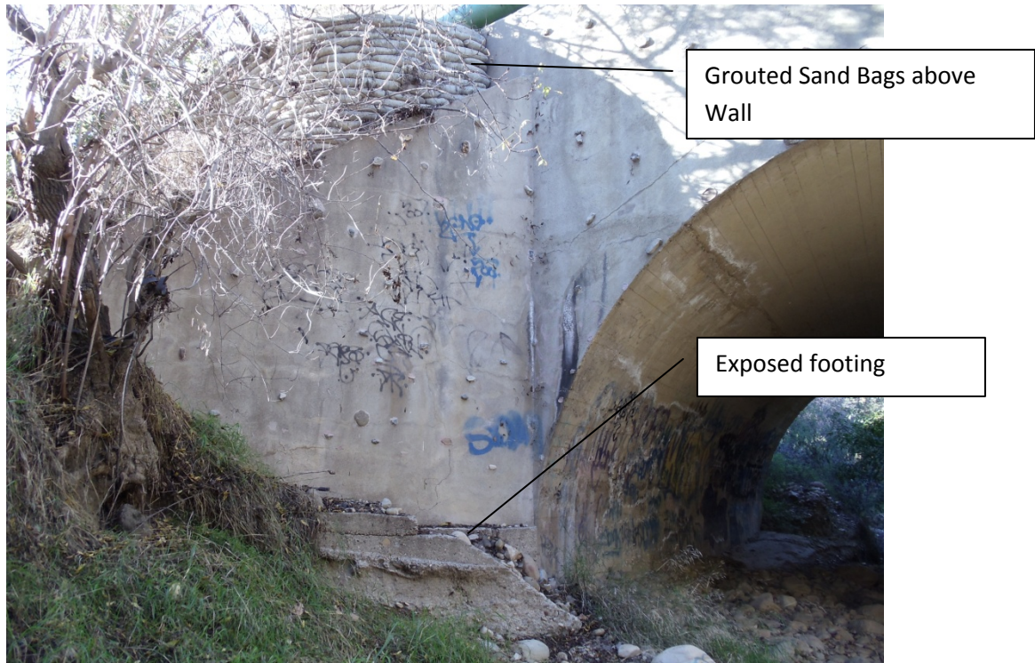
6 Down Stream Wing Wall
