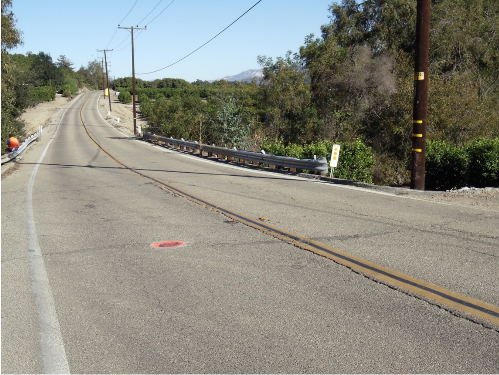
1 Roadway Looking East
