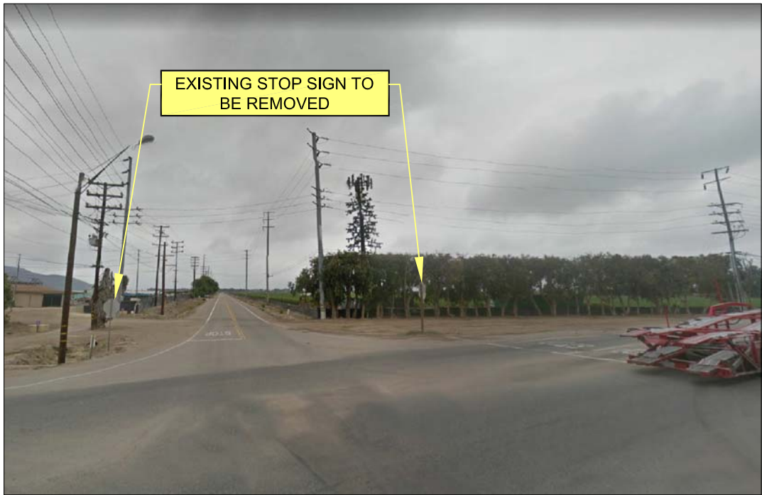
EXISTING CONDITION SOUTHBOUND EXISTING - 4-WAY STOP
