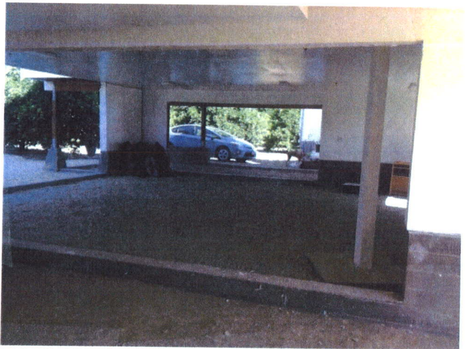
Interior of garage looking north
