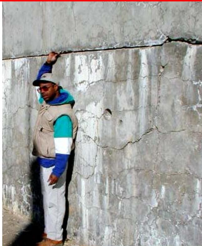
**Figure 1.--Cracked concrete in one 6-ft-tall construction lift, on dam's left half by the powerhouse, close-up (top) and distant views.**
