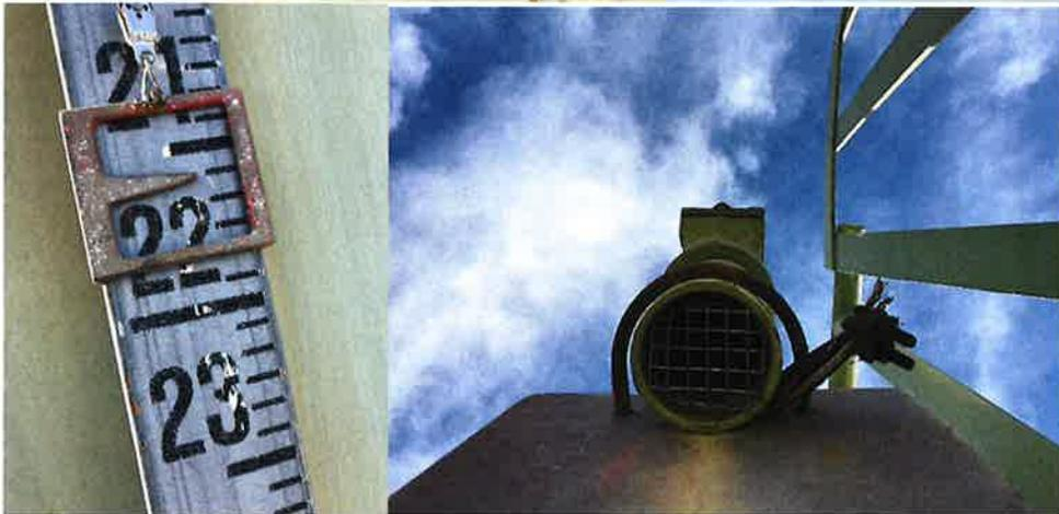
**Response #6:** Greentree Reservoir: Gaps in the screen around the center air vent repaired. Float indicator repaired.
