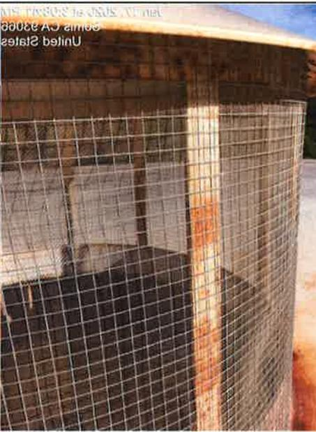
**Response #5:** Balcom Reservoir's vent screen was replaced. Balcom Reservoir, level indicator was removed to avoid false level indication and opening to tank was capped.
