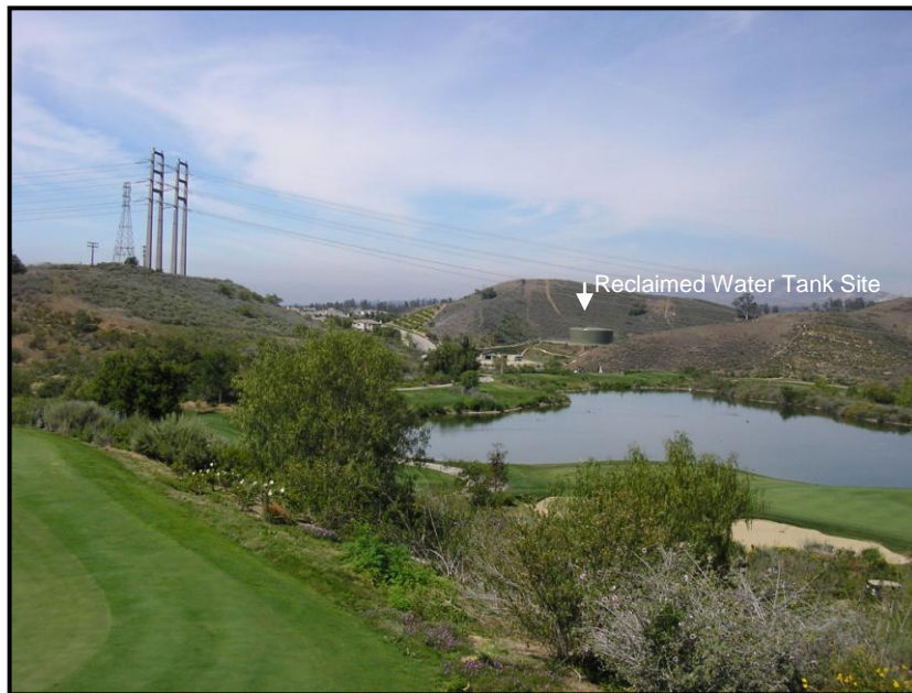
Figure C.6-2. View of Existing Reclaimed Water Tank Site and Well No. 20
